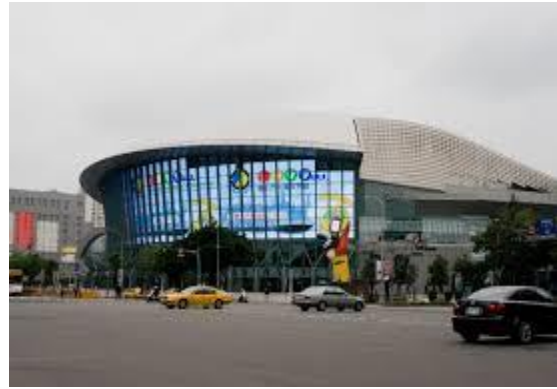
Figure 5: Building integrated LED installation. Source: Wikipedia
